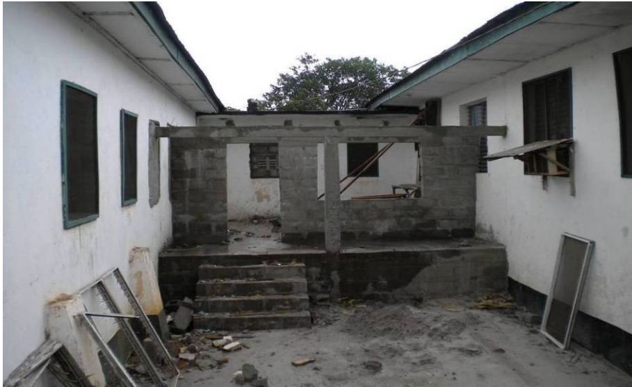
Figure 10-2: Ongoing Infrastructure Rehabilitation Activity at Grand Bassa Government Hospital
